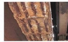
Reinforcement corrosion
