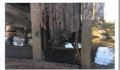
Timber deterioration
