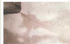
Fatigue cracks on older steel bridges
