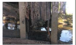
Timber deterioration
