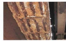
Reinforcement corrosion
